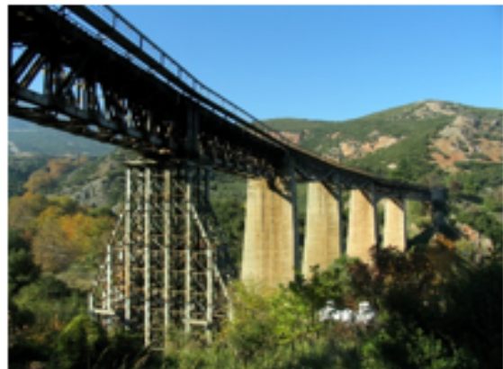
Photo of the GORGOPOTAMOS Bridge. 15 th July 2008 (credit—George Terezakis. Flickr download) (bad seed). Showing the modern replacement of its central span, demolished in "Operation Harling" over 80 years ago.
